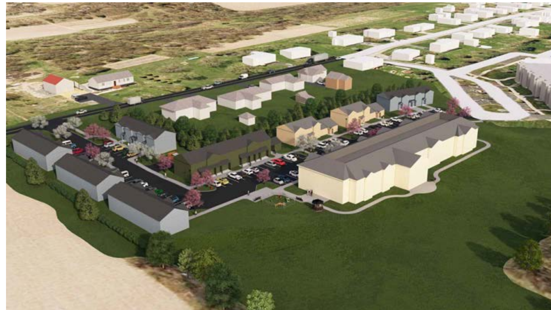
3: LOOKING SOUTHWEST AT PERU ROAD & PROPOSED DEVELOPMENT
