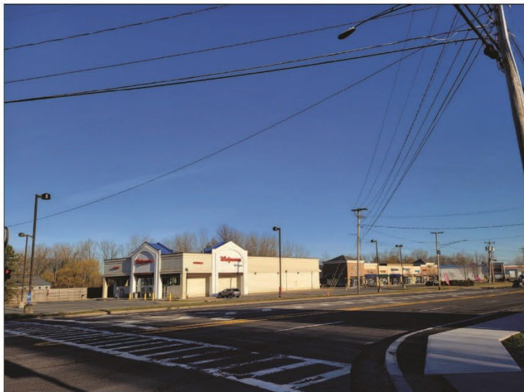
Intersection of U.S Route 11 and Caughdenoy Road
