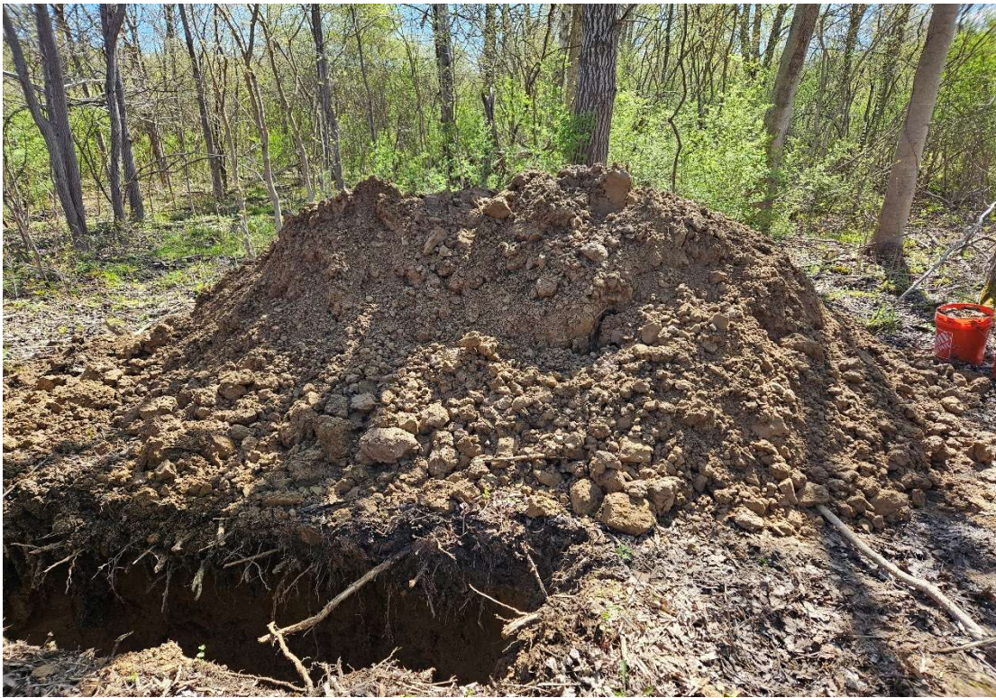
Figure 30: Materials excavated from TP-315
