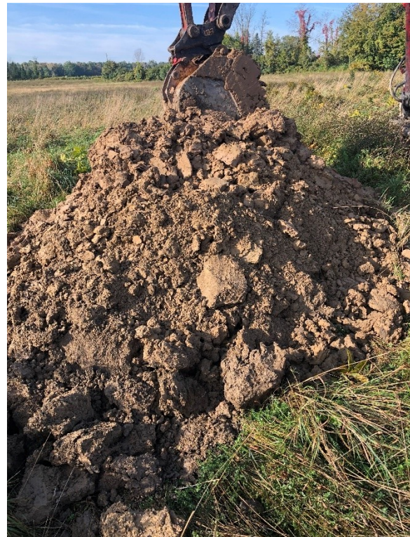
Figure 2: Materials Excavated from Test Pit TP-1
