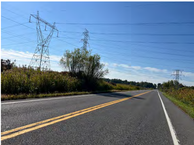
Looking South Along Caughdenoy Road From Northern Boundary
