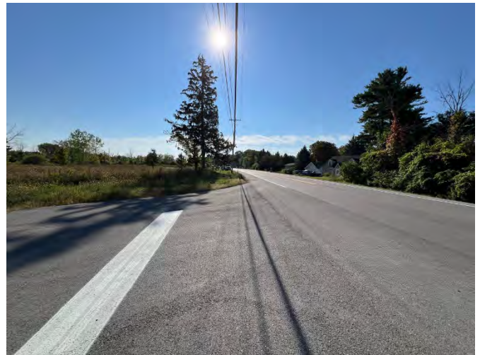
Looking Southeast Along Route 31 From Burnet Road
