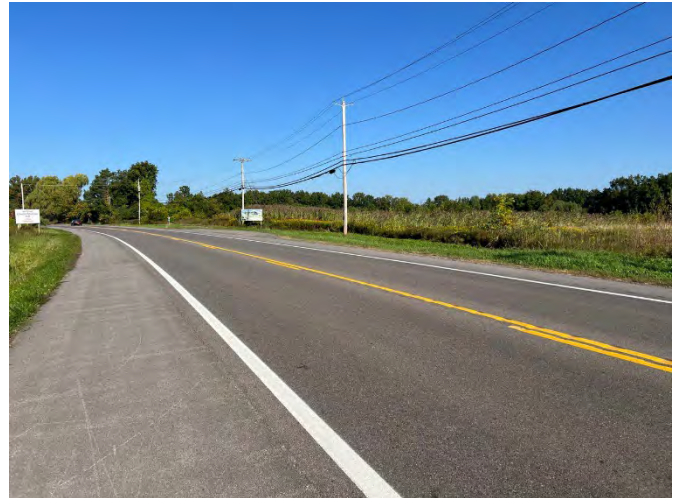
Looking Northwest Along Route 31 Frontage
