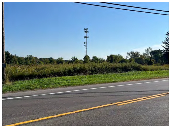
Cell Tower North Of Route 31
