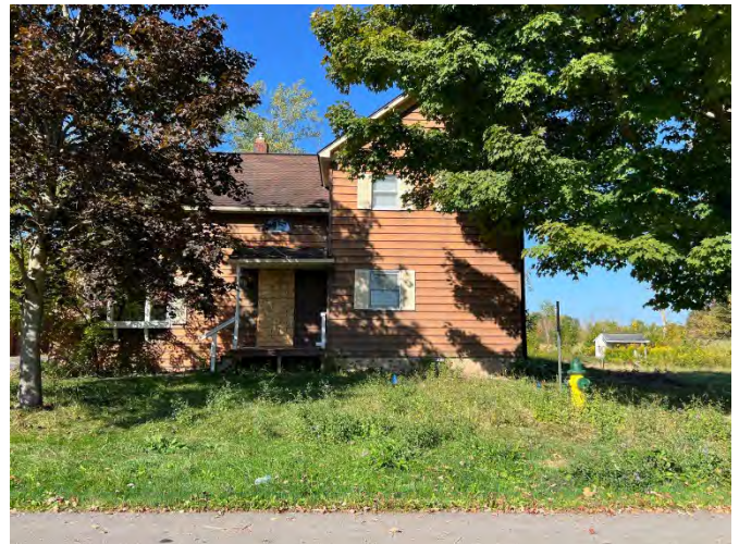
Two-Story House Near End Of Burnet Road
