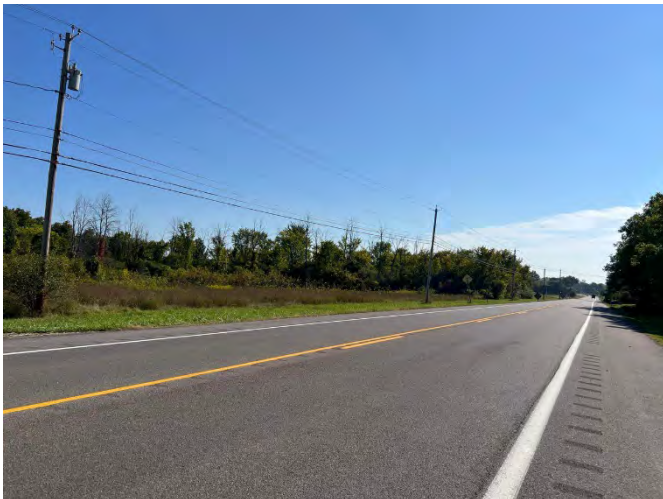
Looking East Along Route 31 East Of Burnet Road
