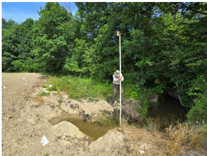
The white wire flags show where rock would be buried to control the head-cut
